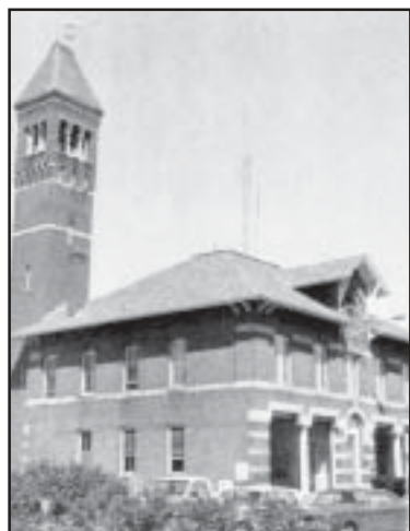
Central Fire Station on Warren Street.
